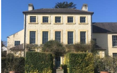
Kildrought House, Celbridge, Co. Kildare Works supported: repairs to garden front windows Grant pledged: €3,000
