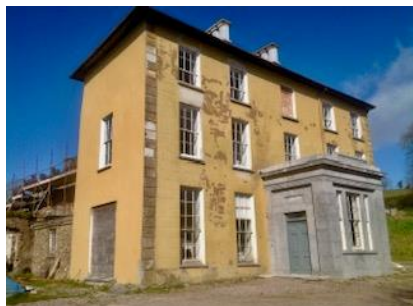
Jamesbrook House, Midelton, Co. Cork Works supported: repair of porch windows Grant pledged: €1,000
