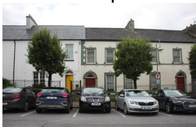
Ivy House, Listowel, Co. Kerry Works supported: damp control Grant pledged: €1,000
