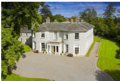
Kilsharvan House, Bellewstown, Co. Meath Works supported: window repairs Grant pledged: €3,000
