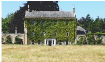
Killyon Manor, C. Meath Works supported: roof repairs to ballroom Grant pledged: €2,500
