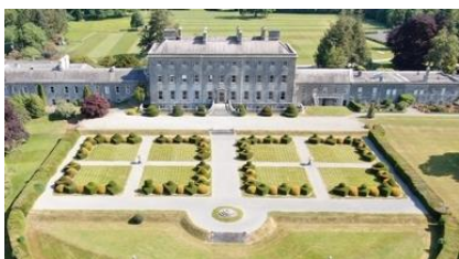
Headfort House, Kells, Co. Meath Works supported: sash window repairs Grant pledged: €3,000
