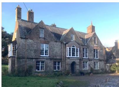
Myrtle Grove, Youghal, Co. Cork Works supported: window repairs Grant pledged: €3,000
