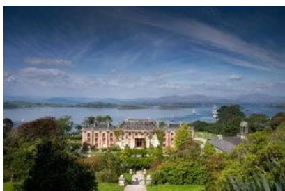
Bantry House, Bantry, Co. Cork Works supported: Roof repairs and doors to basement Grant pledged: €3,000
