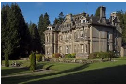
Clonalis House, Co. Roscommon Works supported: window repairs Grant pledged: €2,500
