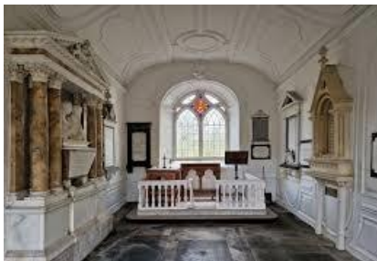
Fiddown Church, Co Kilkenny Works supported: Repairs to roof and rainwater goods Grant pledged: €2,500
