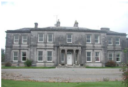
Annaghmore House, Co. Sligo Works supported: window repairs Grant pledged: €3,000
