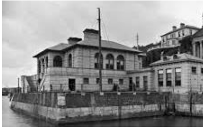
Sirius Arts Centre, Cobh, Co. Cork Works supported: underpinning of loggia Grant pledged: €3,000
