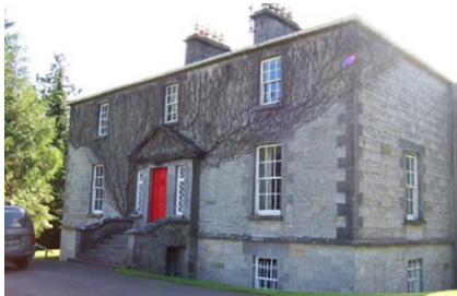
Toberfeckin House, Co. Sligo Works supported: Pediment repairs Grant pledged: €2,000
