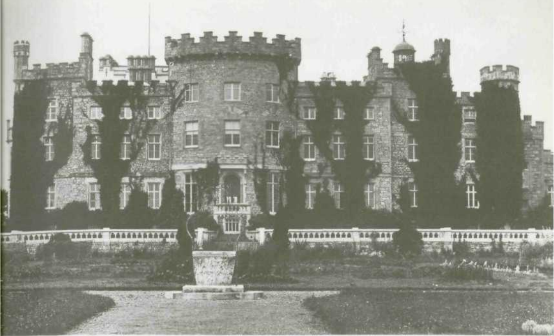
18. Markree Castle, view of south-east elevation (Lawr. Coll.).
