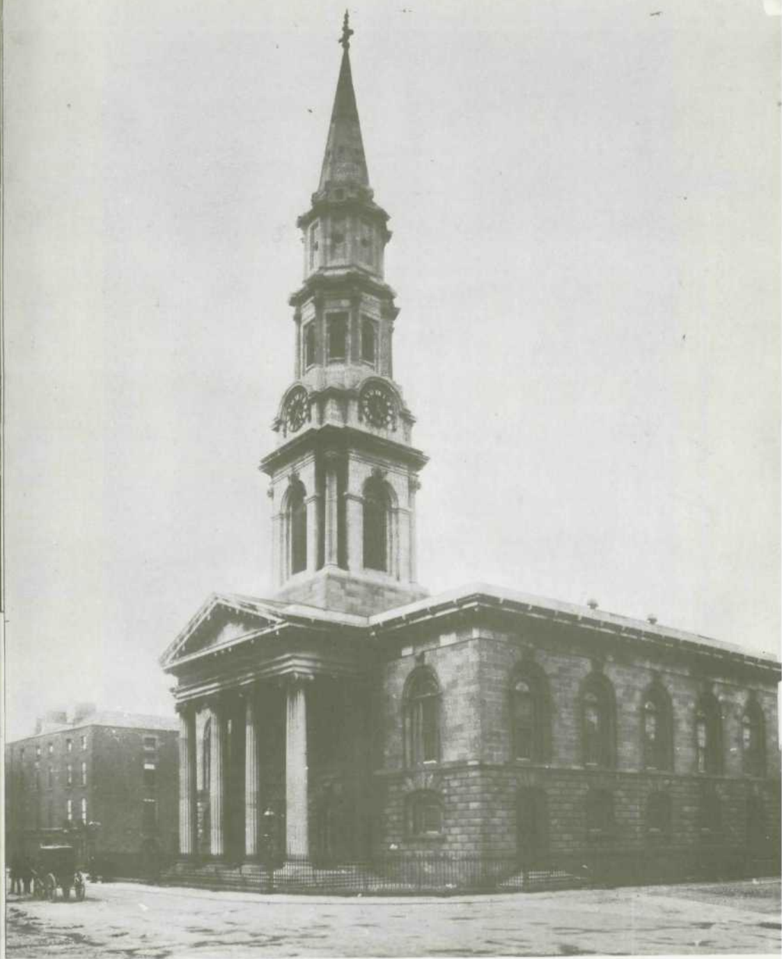
34. St. George's Church, Dublin, view from Temple Street.
