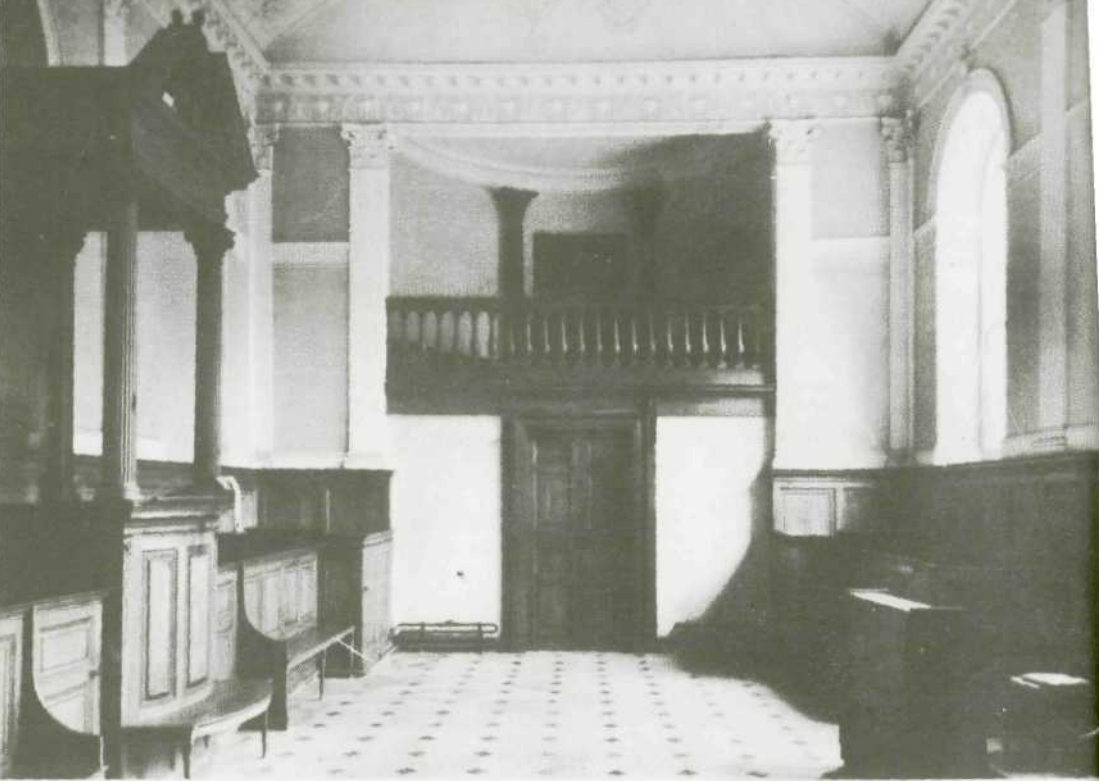
27. Primate's Chapel, view of west end.
