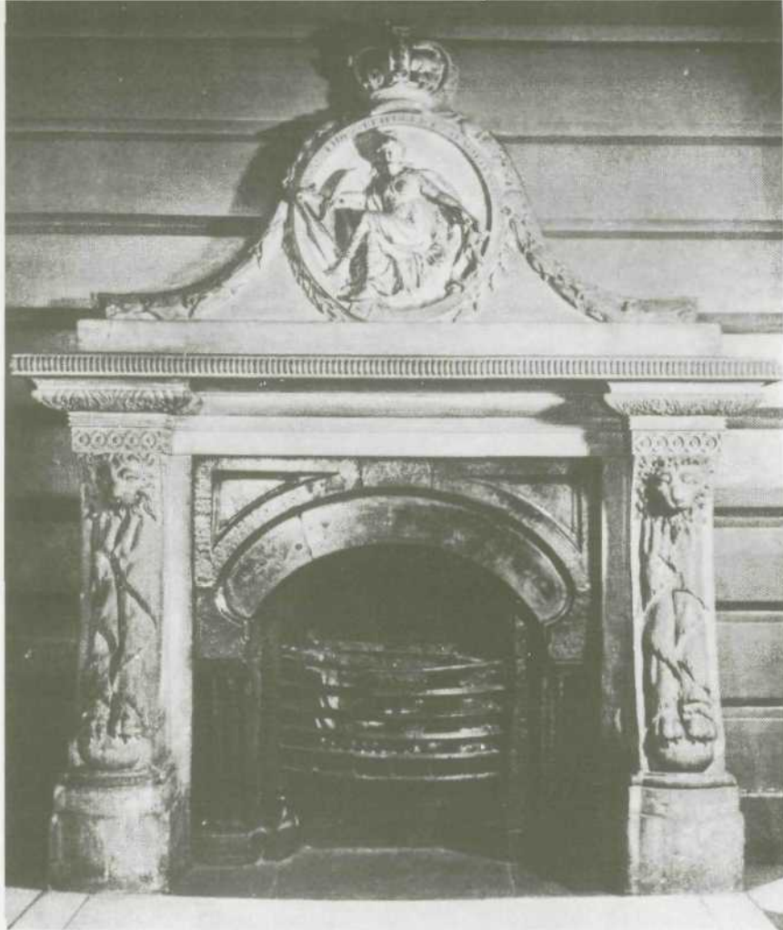
47. Bank of Ireland, Chimney piece in West Hall, probably executed by Thomas Kirk from Francis Johnston's designs.
