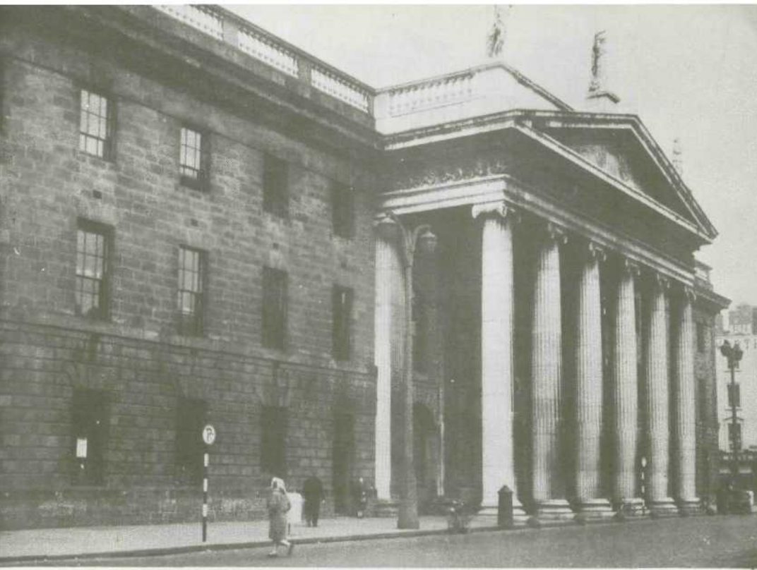
52. General Post Office, Dublin, view of east elevation.
