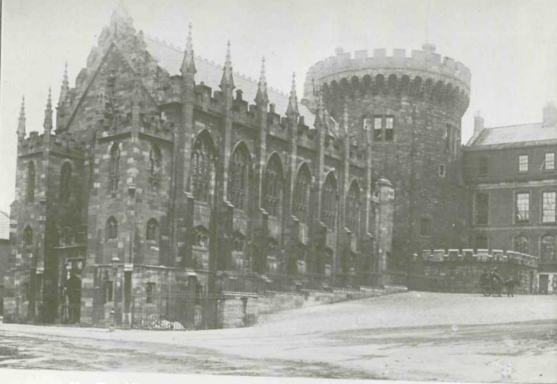
31. Chapel Royal, Dublin Castle, view of north elevation (Lawr. Coll.).
