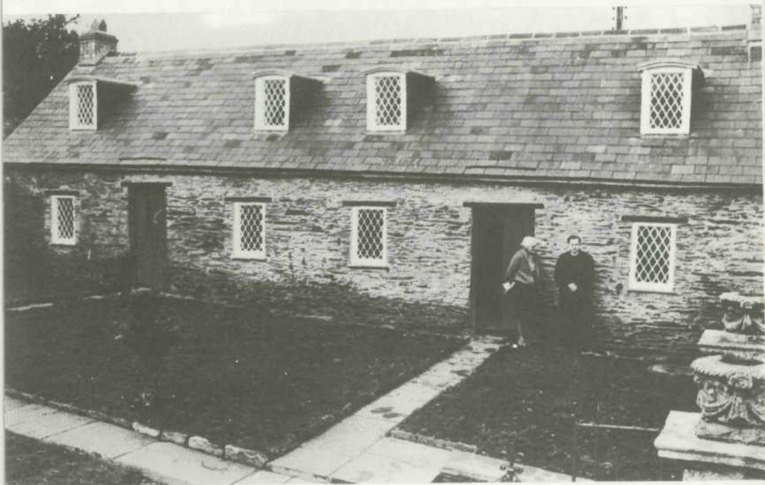
Two of the Gift Houses, Kinsale, after restoration. They were opened by An Taoiseach in 1968.
