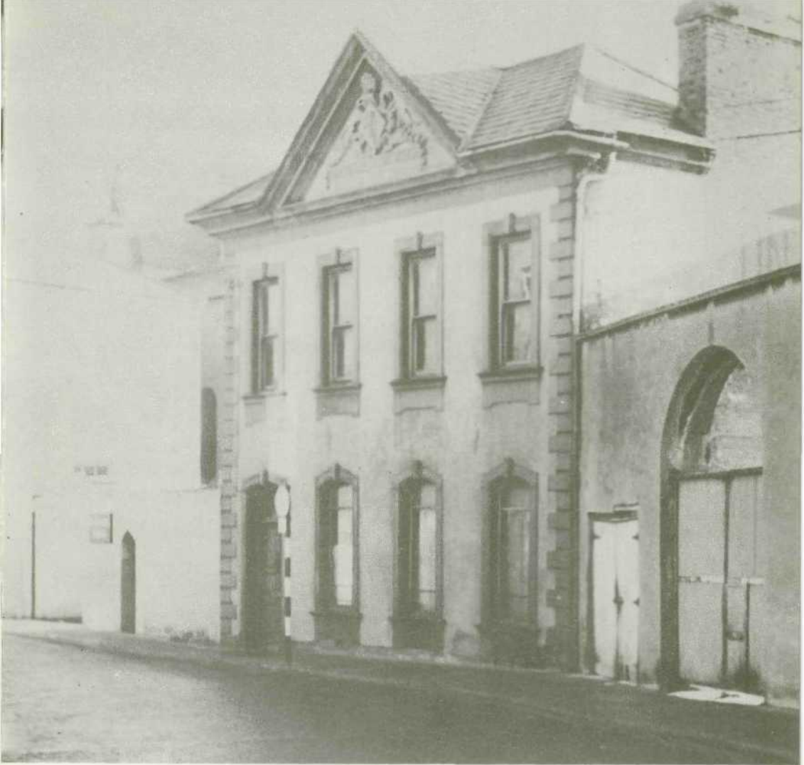
Plate 26. MARY MASON'S SCHOOL, WATERFORD (1740). The Irish Georgian Society has offered to restore the facade of this little masterpiece if it is spared from demolition. Paint must be removed from the stone quoins and the plaster taken off the brick.
