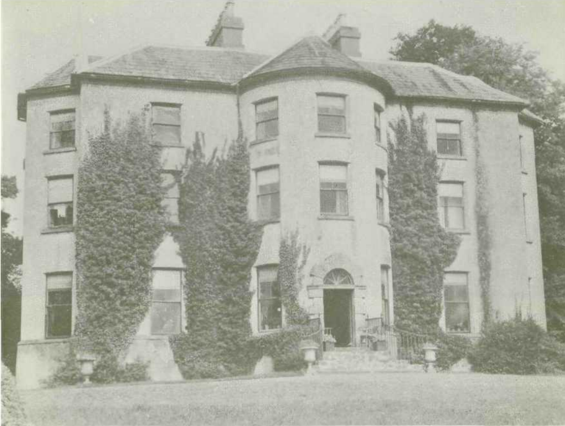
Plate 22. LONGFIELD HOUSE, GOOLDSCROSS, CASHEL, CO. TIPPERARY, Bianconi's home, partially restored in 1967, will be open to the public this year.
