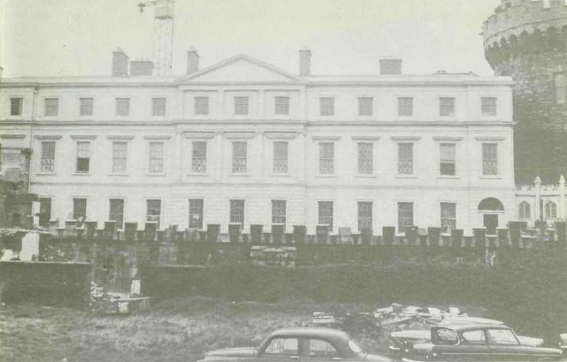
Plate 18. DUBLIN CASTLE. A magnificent job has been made of re-facing the Garden Front of the Castle, under the supervision of Oscar Richardson, Architect, Board of Works.
