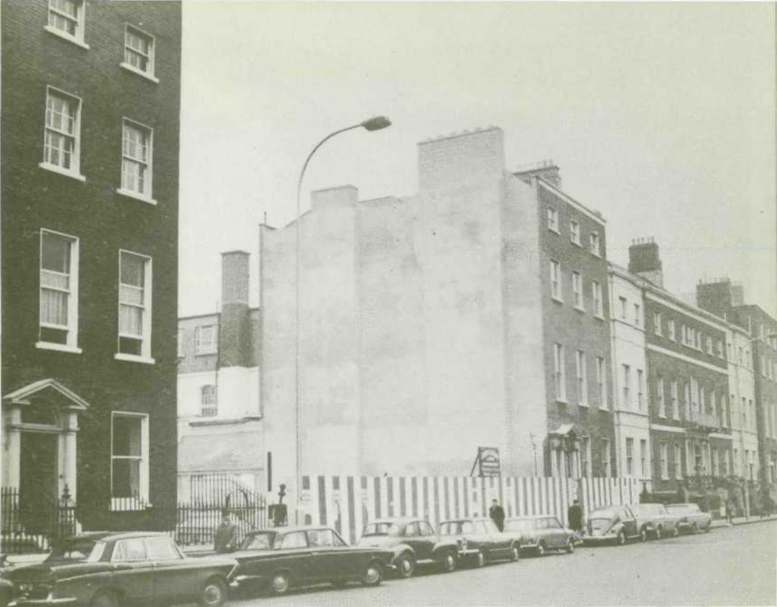
Plate 10. ST. STEPHEN'S GREEN showing the gap where Green Properties Ltd. hastily demolished three houses.
