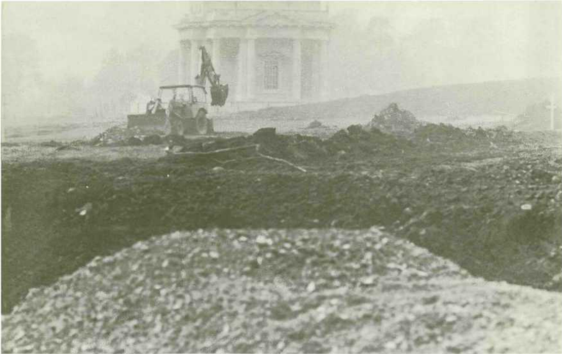
Plate 9. BULLDOZERS creeping up on the Marino Casino.
