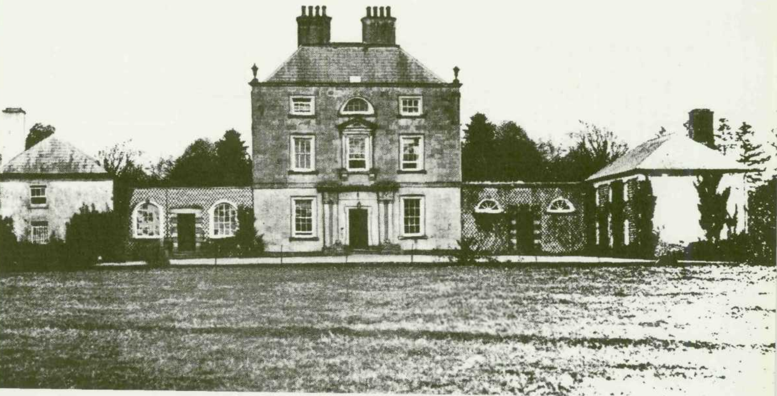
Plate 1. Furness, Co. Kildare. This photograph has been altered to exclude the later additions over the left hand wing. (Reproduced from Sadleir and Dickinson's Georgian Mansions in Ireland , plate LXII.)
