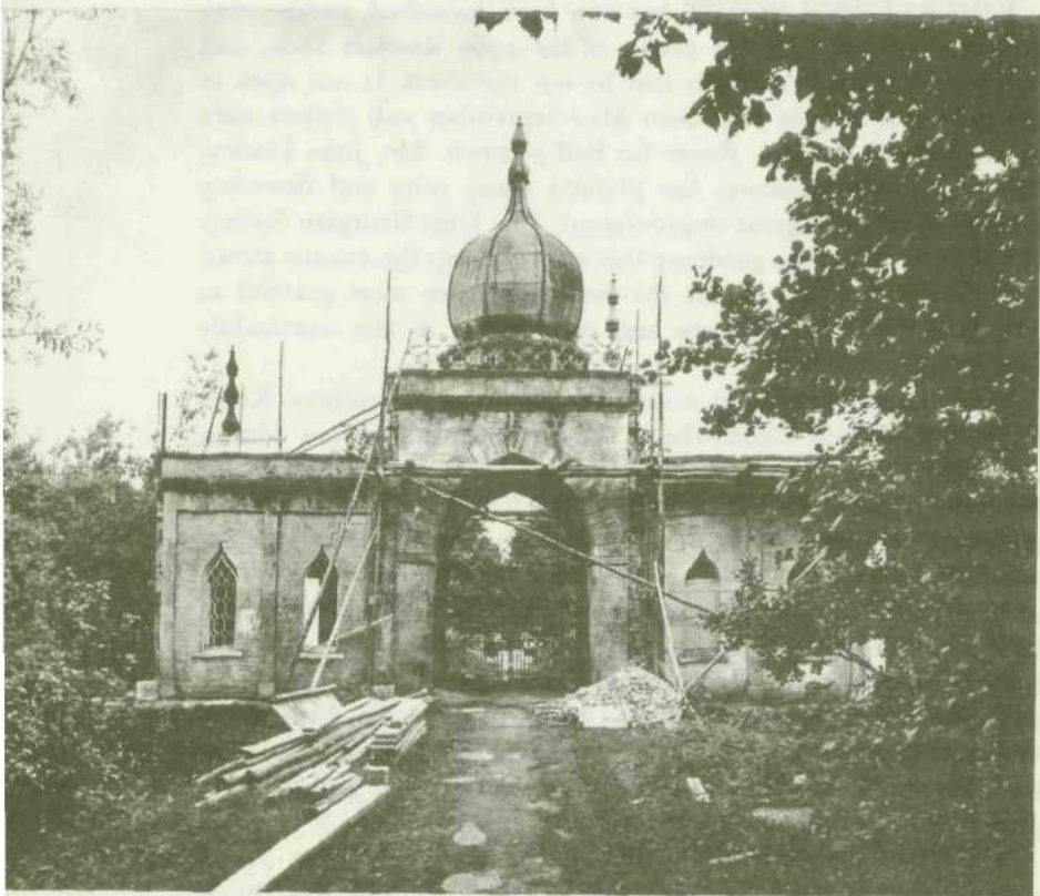
Restoration work at Dromana, July 1966.
