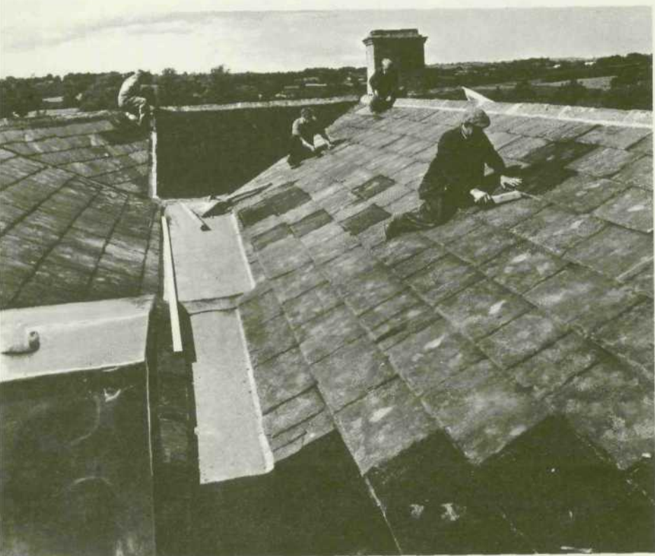
Work on the roof at Gill Hall, Dromore, Co. Down, June 1966.
