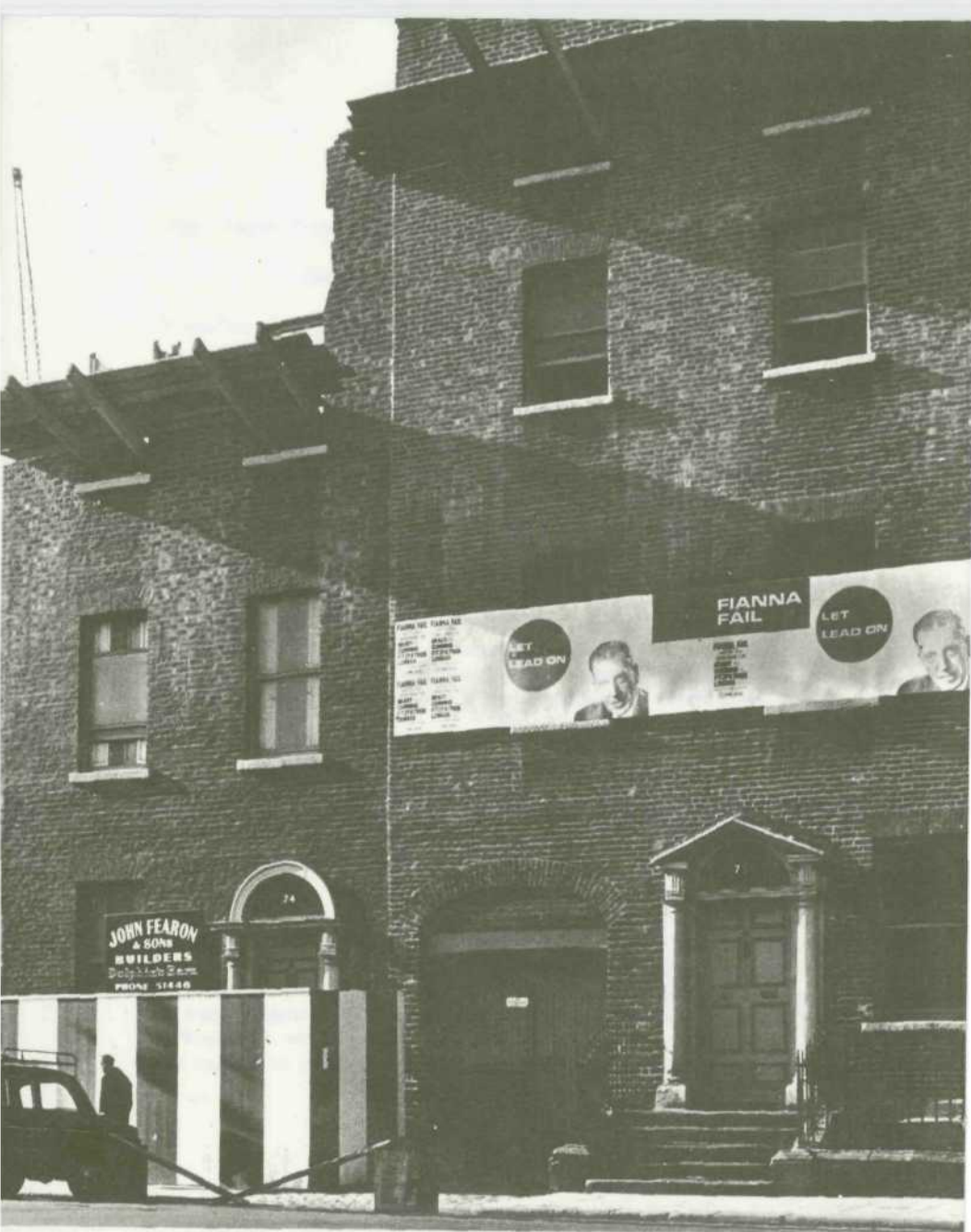
St. Stephen's Green, Dublin, 1965—the wreckers at work. Photo: Green Studio
